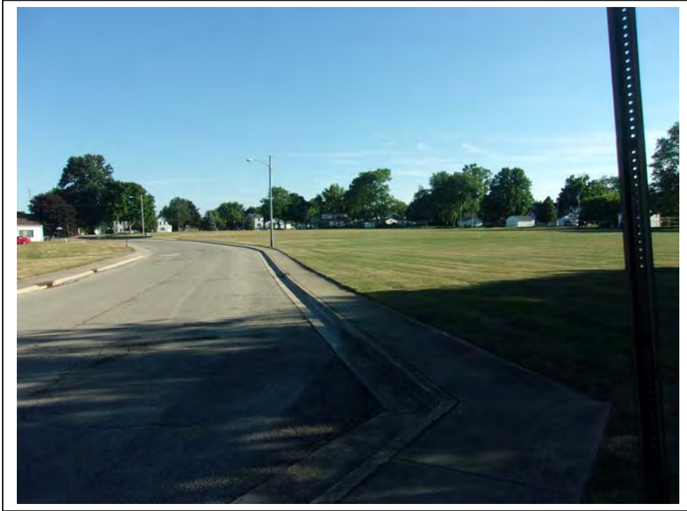
LOOKING SOUTH ALONG FORD DRIVE ALONG EAST PROPERTY LINE
