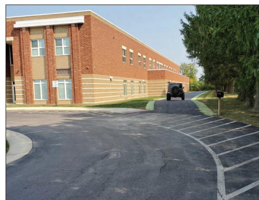
A new road at Springcreek allows for parents to wait on school property vs. on St. Rt. 36, making pick-up and drop-off times safer.
